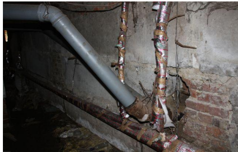
7.) pipes in underground floor
