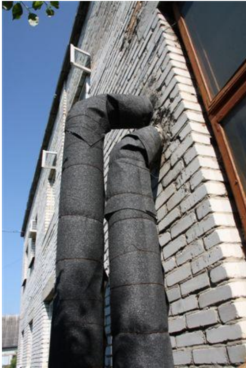
13.) piping insulation
