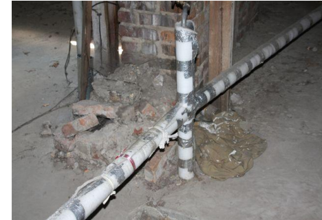
3.) piping insulation on roof
